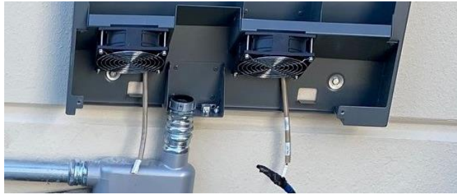
Conduit Install shown as a comparison
