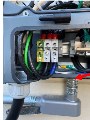
Conduit Installation 1.25" secured to bottom mounting area. 1-phase Version Shown
