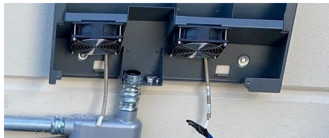
Conduit Install shown as a comparison
