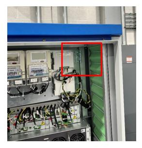
• Prior to drilling the roof hole for this procedure. You must place a catch for the debris that will form while drilling in the location marked by the red square.
