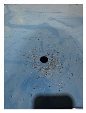
Use a 7/8in Uni Bit to drill all the way through where the pilot hole was made.
