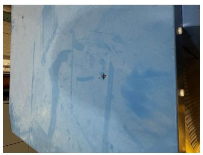
• Once you measure out the location of where the hole will be drilled out. Mark it on the top blue roof of the charger.
