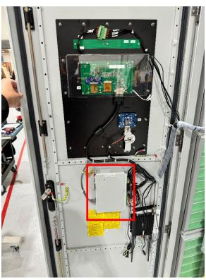
Run the Black (MU-J13-7/485-B) and White (MU-J13-5/485-A) wires to the IMMU2 Located on the front door.
