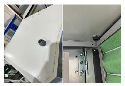
■ Take the ½" Nylon Liquid Tight Fitting Type B and install it in the orientation shown in the pictures above. Tighten the seal nut from inside of the charger.
