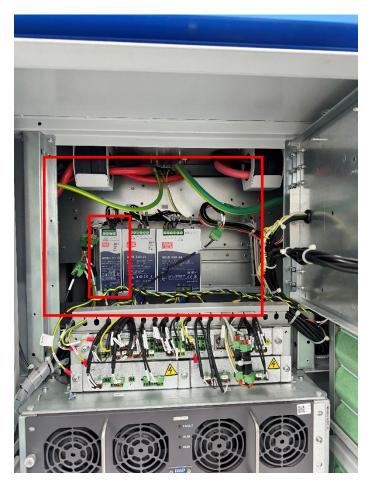
After splicing the main wire harness, Run the Red (LU-J1-2/12V+) and Green/Yellow (LU1-J1-3/GND) wires behind the small upper door shown in the image to land in the 12V Auxiliary power shown above.
