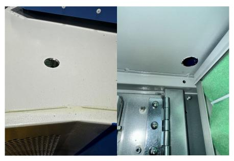
• After drilling the pass-through hole. Remove the blue cover and clean up all metal debris that may still be there.
