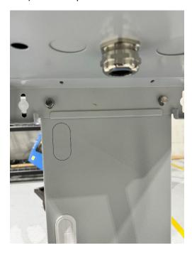
On the bottom bracket, locate the last two mounting holes and use the two M10\*30 bolts to secure the EVSE bracket in place.
