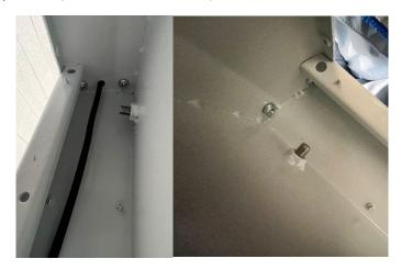
With the wire successfully ran through the pedestal. Insert the four M8\*20 bolts to connect the two pieces together.
