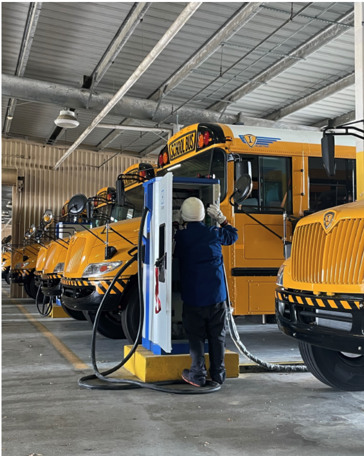
InCharge technician servicing an ICE-60 DC Fast charger.
