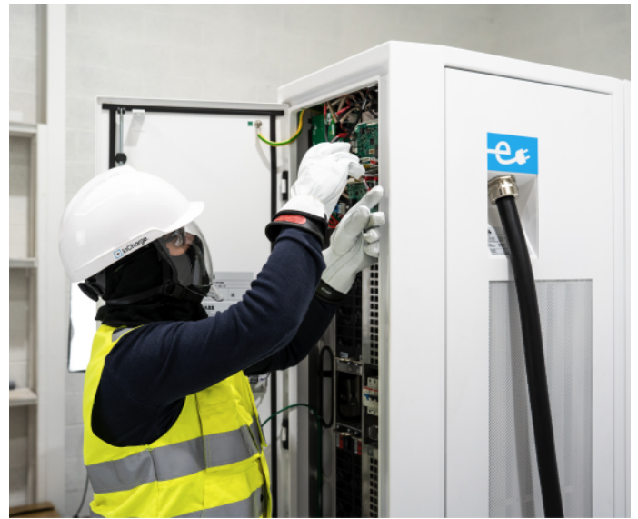
InCharge technician servicing an ABB Terra DC Fast charger.
