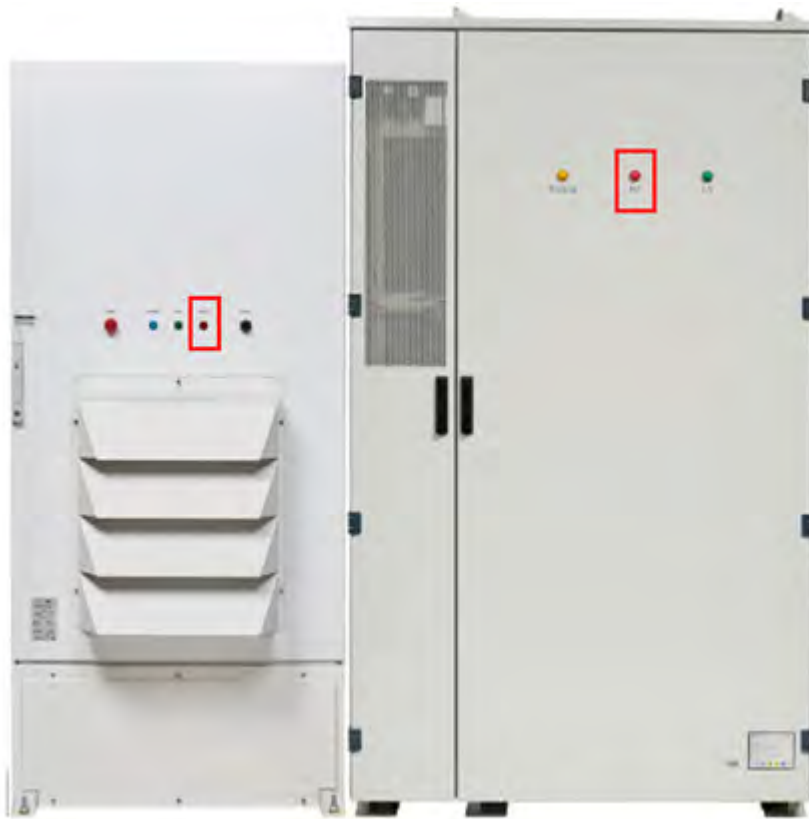
Figure 71. Inverter and Battery Run Indicator Locations
